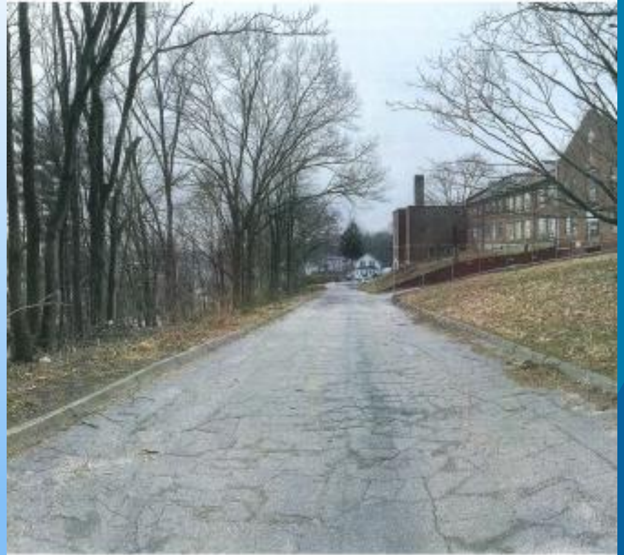
GLADSTONE ELEMENTARY SCHOOL EAST FACADE - VIEW TO SOUTH ALONG ACCESS DRIVEWAY
