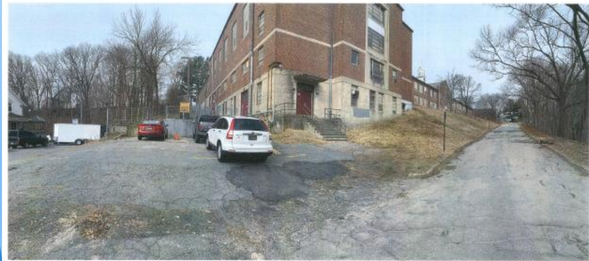
GLADSTONE ELEMENTARY SCHOOL SOUTH & EAST FACADE - VIEW TO NORTHWEST FROM ACCESS DRIVEWAY
